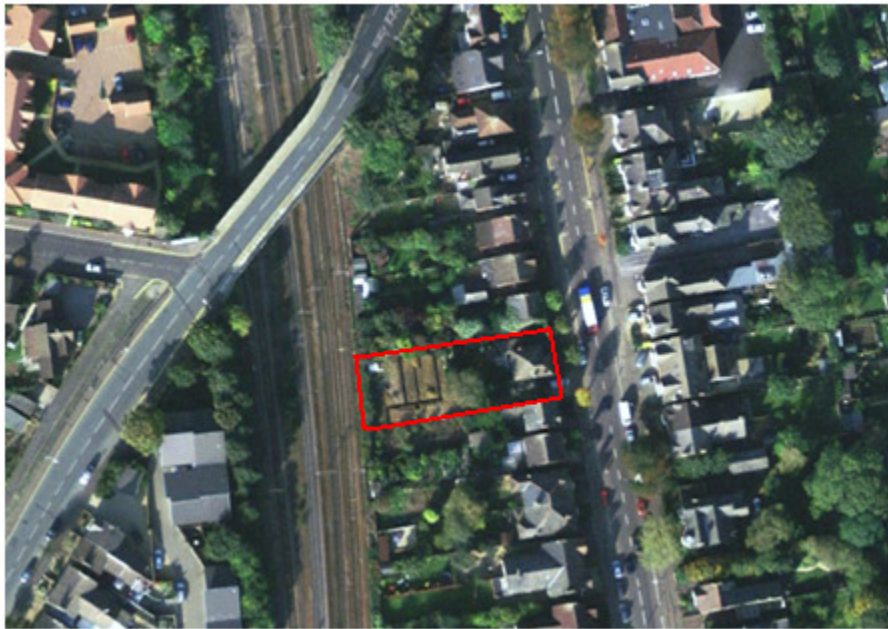
Fig 07: Showing the rear of 22 Fletton Avenue with foundations in for development
